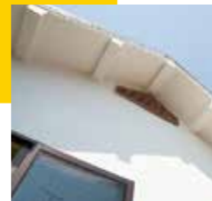
屋根・外壁 Roof & Outer wall
